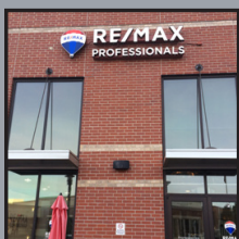
DENVER TECH CENTER
