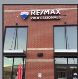
DENVER TECH CENTER
